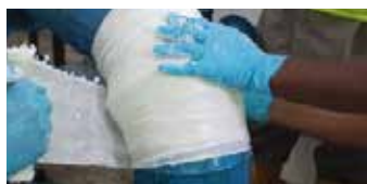
INSTANT LIVE LEAK PIPELINE REPAIR
