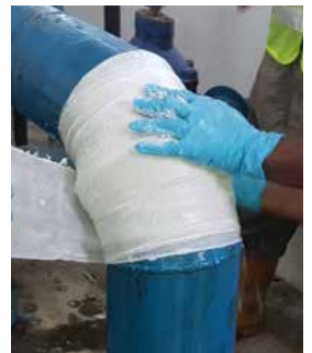
INSTANT LIVE LEAK PIPELINE REPAIR
